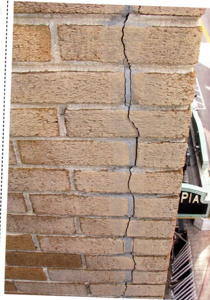
Diagonal brick cracking originating from the lintel ends.
