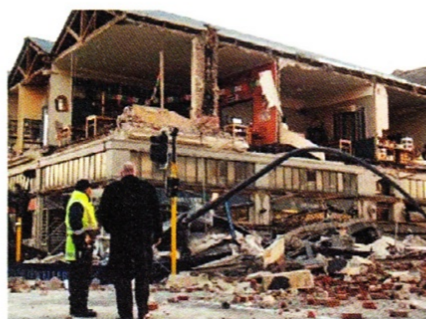
Earthquakes magnify any inherent faults in a building's original design.
