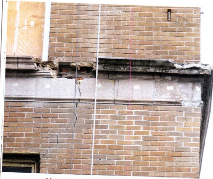
Diagonal brick cracking originating from the lintel ends.
