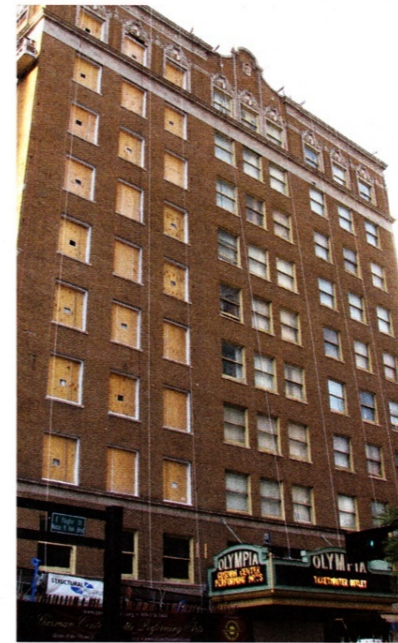
Sections of the Olympic Theater (Miami) were taken down and rebuilt to address structural and safety issues.
